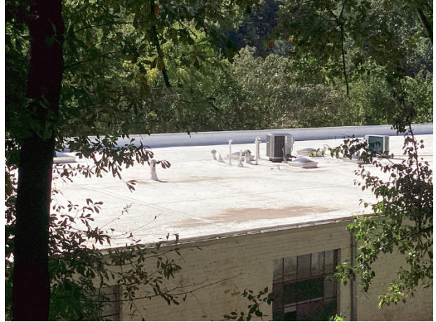
Evidence of standing water at building 4
