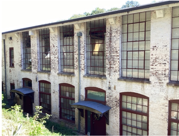
Original factory steel window frames
