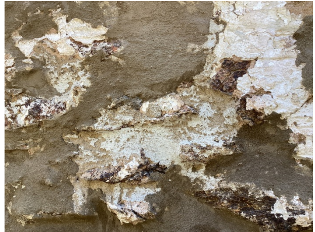
Detail view of River rock and mortar
