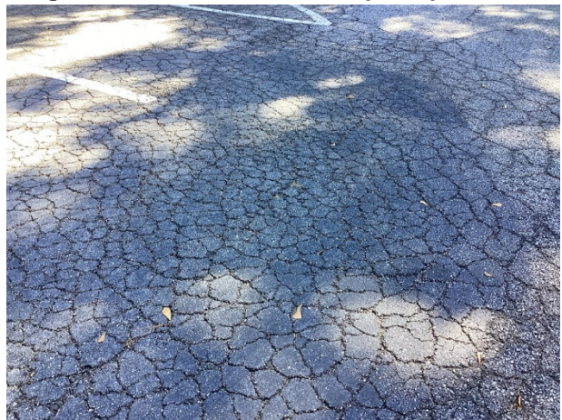
Alligator cracks at upper parking area
