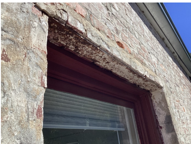
Significantly weathered lintel
