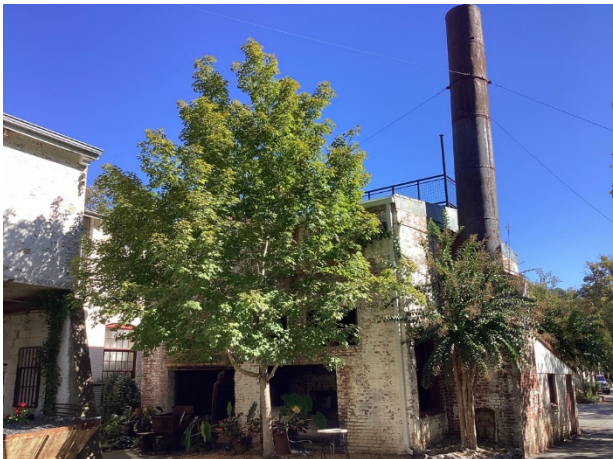
Historic mill equipment house, note chimney stack secured with cables
