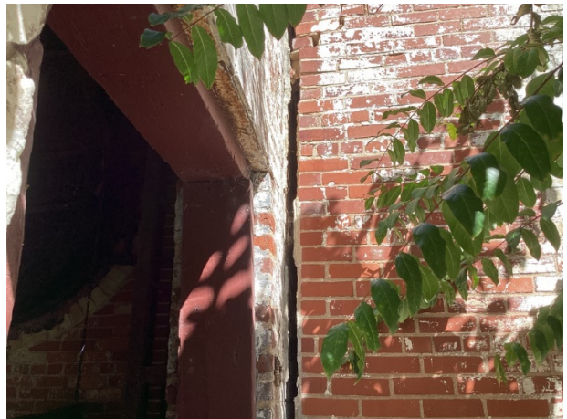
Separation at chimney joint at historic equipment house
