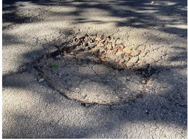
Significant deterioration of asphalt pavement
