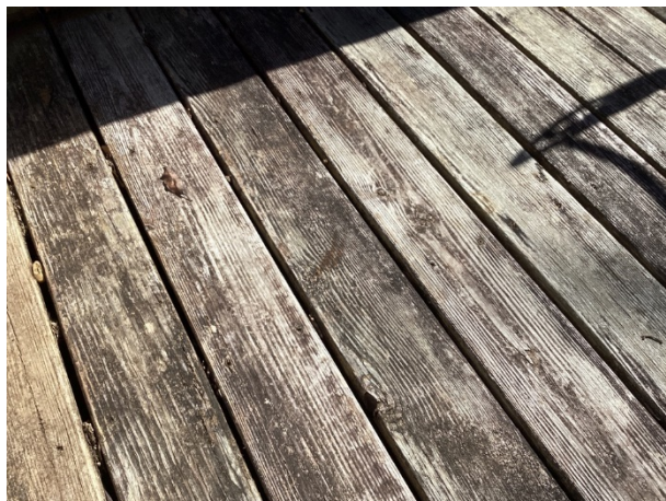
Weathered wood decking
