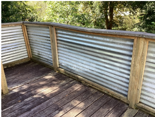
Galvanized steel and wood railing
