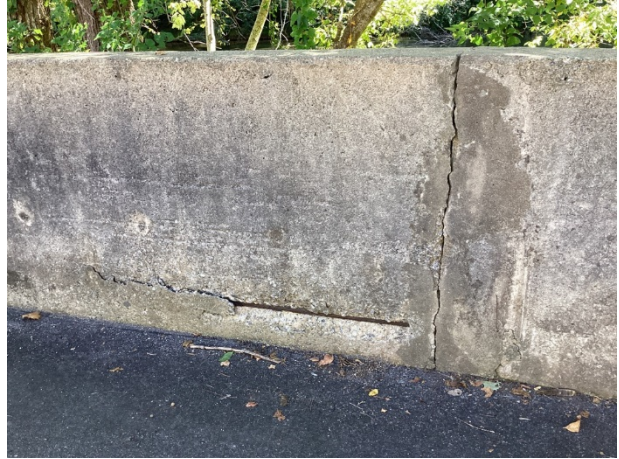
Cracks and exposed concrete reinforcement
