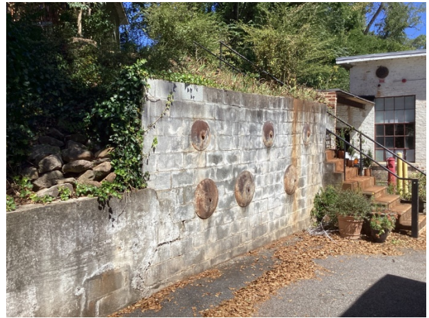
Stabilized retaining wall with repairs
