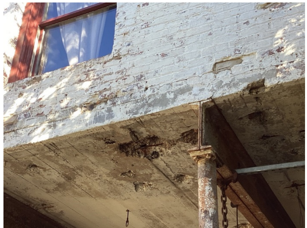
Masonry cracks and concrete deterioration with exposed reinforcement
