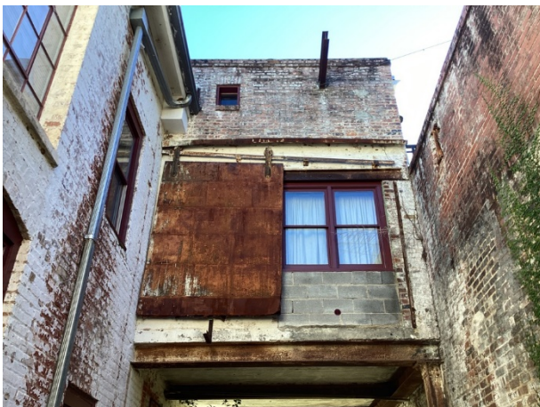
Weathered masonry with partial replacements at unit 5
