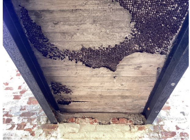
Catwalk unit 31 (Note exposed concrete reinforcement)
