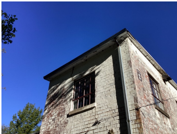
Galvanized gutters and downspouts
