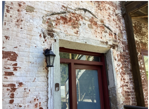
Significant masonry repairs at doorway
