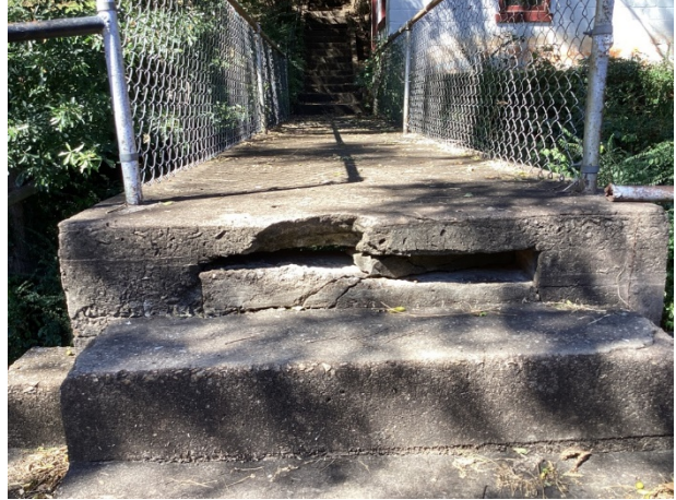
Deterioration at concrete stairs at pedestrian bridge
