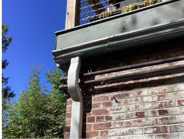
Galvanized and aluminum gutters and downspouts
