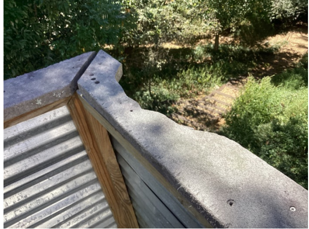
Damaged composite railing
