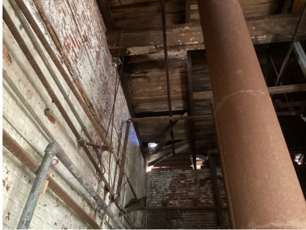
Significant wood deterioration at underside of roofing system at historic mill equipment
