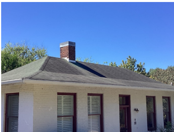
Weathered three-tab shingles at building 3
