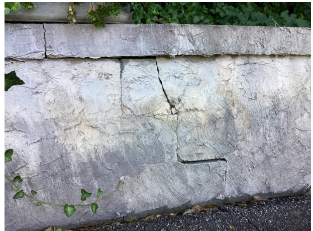
Step cracks and header deterioration
