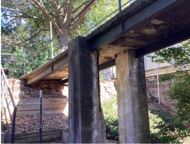
Catwalk at unit 31 (Note exposed concrete reinforcement at column)
