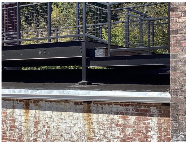
Modified bitumen roof system beneath deck at historic equipment house
