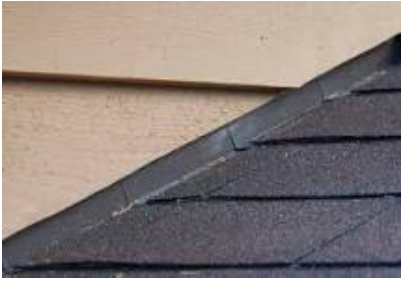
Stock image of proper step flashing
