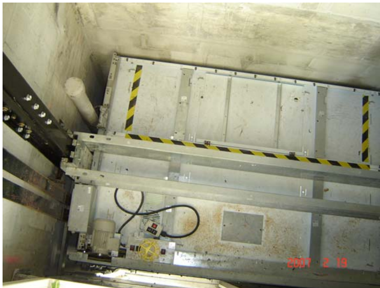
LOW RISE PARKING GARAGE/TENNIS DECK HYDRAULIC ELEVATOR HOISTWAY VIEW SHOWING TOP OF CAR, DOOR OPERATOR, GUIDE RAILS, DUAL JACK HOLELESS HYDRAULIC JACKS, INSPECTION OPERATION CONTROLS, ETC.
