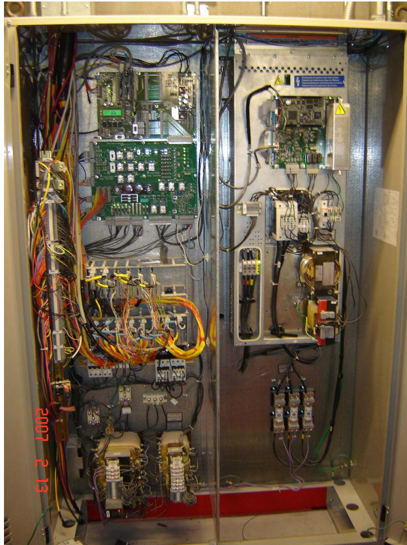
HIGH RISE PASSENGER ELEVATOR VIEW OF MICROPROCESSOR BASED TRACTION ELEVATOR CONTROL SYSTEM WITH DIGITAL DRIVES.
