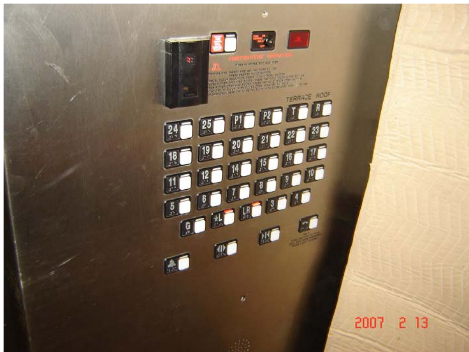
VIEW OF HIGH RISE PASSENGER CARS PE1-PE10 CAB WITH STANDARD CAR FIXTURES.
