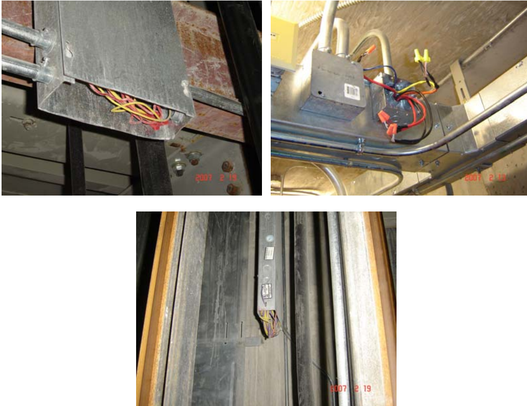
VIEW OF TYPICAL MISSING COVERS ON WIRING BOX/DUCT IN HIGHRISE MACHINE ROOM/HOISTWAY THAT NEEDS TO BE REPLACED.
