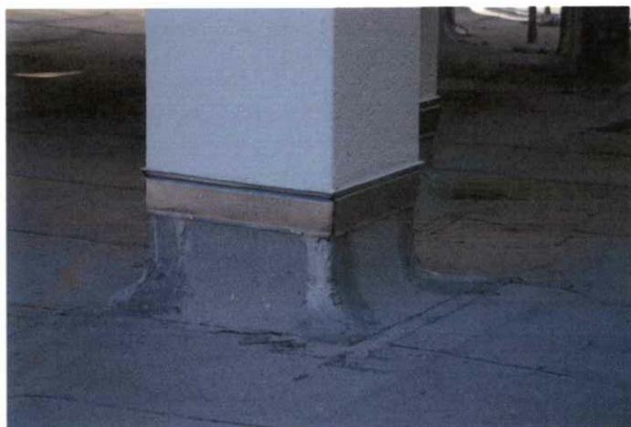
Proper Corner Flashing
