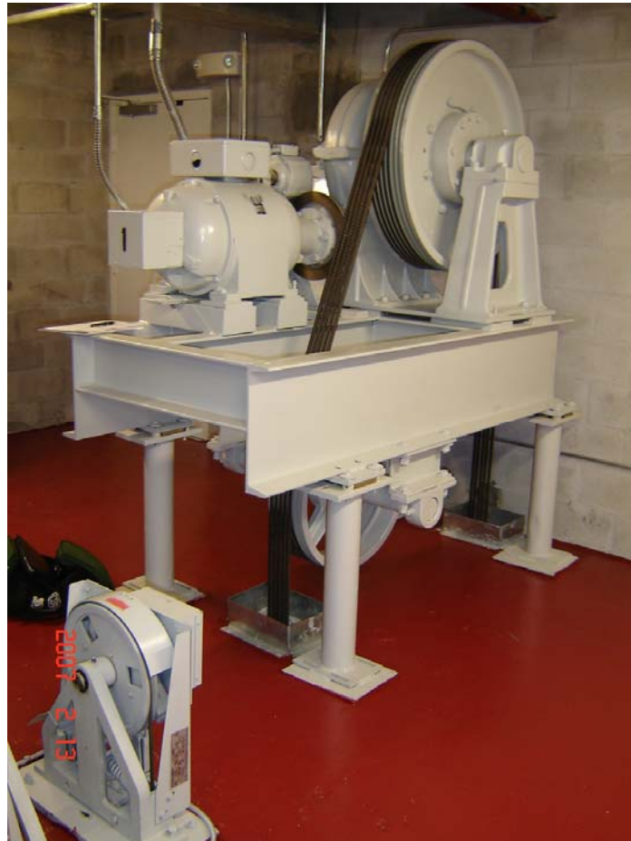
HIGH RISE PASSENGER ELEVATOR MACHINE ROOM VIEW OF OVERHEAD GEARED TRACTION HOIST MACHINE, MOTOR, BRAKE, DRIVE/DEFLECTOR SHEAVES & OVERSPEED GOVERNOR.
