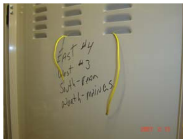
VIEW OF TEMPORARY JUMPER WIRES THAT MUST BE REMOVED FROM BUILDING TO PREVENT UNSAFE OPERATION OF ELEVATORS.
