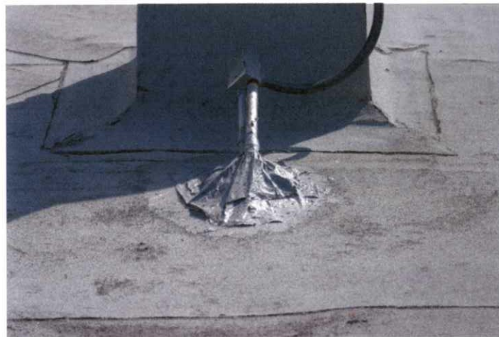
Missing Pitch Pan (must be replaced)
