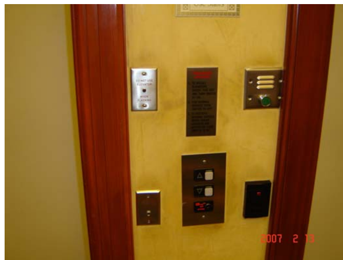
VIEW OF TOWER HIGH RISE PASSENGER CARS PE1-PE10 MAIN LOBBY (TOP) AND CLOSE UP OF STANDARD HALL BUTTON FIXTURES (BOTTOM.)
