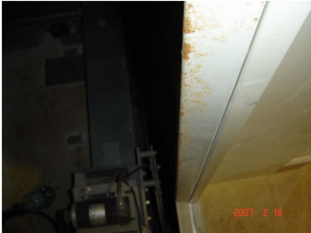
TYPICAL VIEWS OF RUST DEVELOPING ON ELEVATOR ENTRANCE EQUIPMENT REQUIRING CORRECTION TO PREVENT FURTHER DAMAGE.
