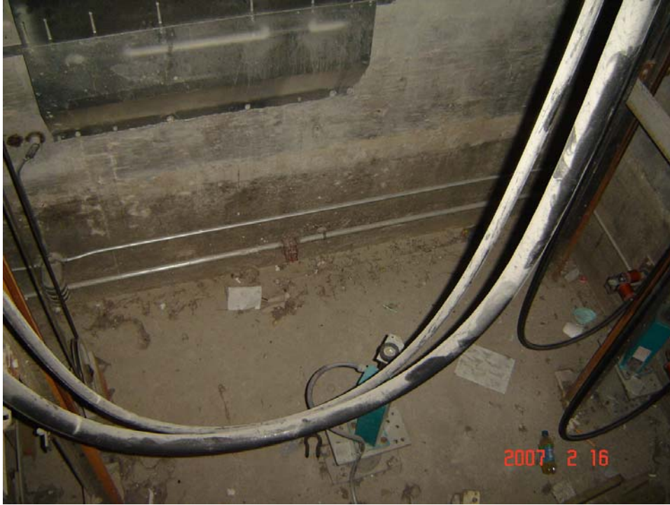
HIGH RISE PASSENGER TRACTION ELEVATOR HOISTWAY PIT VIEW OF OIL BUFFER, GOVERNOR SHEAVE, GUIDE RAIL, COMPENSATION, ETC.
