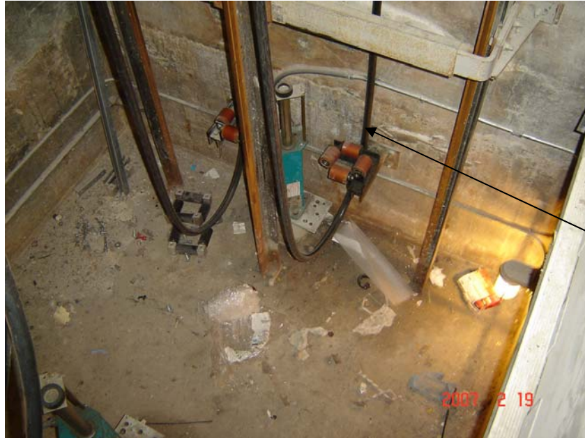
VIEW OF HIGH RISE ELEVATOR PE6 COMPENSATION CABLE SHOWING HOW CABLE IS NOT IN CENTER OF FOUR GUIDE ROLLERS.
