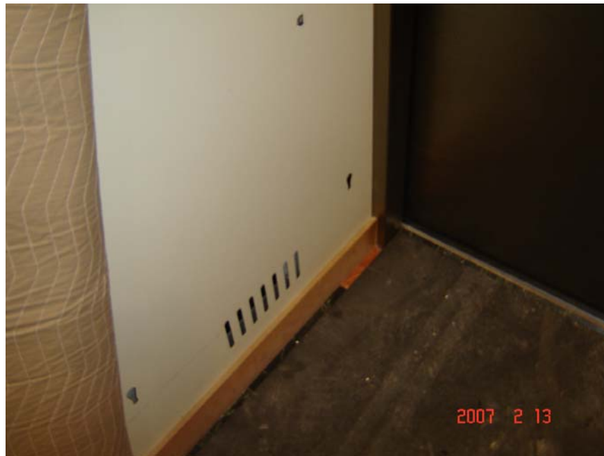
TYPICAL VIEWS OF UNFINISHED CAB INTERIORS SHOWING SHELL CAB WALL (WHITE) INSTEAD OF MOSTLY FINISHED INTERIORS. THIS CONDITION IS ON THE "CONTRACTOR CARS" PE2, PE4, PE6, PE8, PE10 IN EACH CORE OF THE BUILDING.
