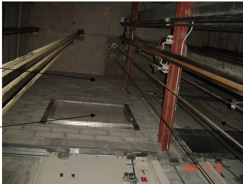
VIEW OF TYPICAL HIGH RISE ELEVATOR HOISTWAY VENT. NOTE LOCATION NEXT TO ROOF FLOOR ELEVATOR DOOR INSTEAD OF CODE REQUIRED LOCATION AT TOP OR HOISTWAY JUST UNDER MACHINE ROOM SLAB. MUST BE INVESTIGATED FOR CONFORMANCE/APPROVAL.
