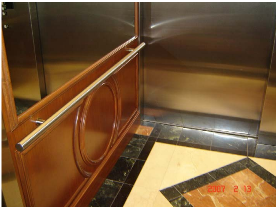
VIEW OF HIGH RISE ELEVATORS PE1-10 CAB INTERIOR FINISHES SHOWING CEILING/WALLS/DOORS (TOP) AND WALLS/LOWER/BASE/FLOOR (BOTTOM) MOSTLY FINISHED ONLY ON "RESIDENT CARS" PE1, PE3, PE5, PE7, PE9.
