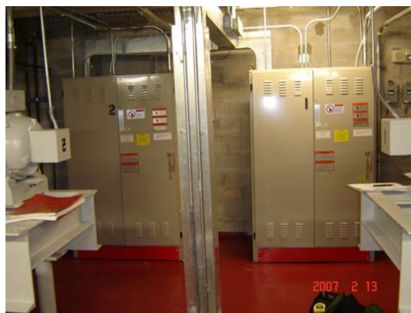
HIGH RISE ELEVATOR MACHINE ROOM VIEW OF CONTROLLERS.
