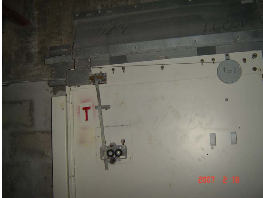
TYPICAL VIEW OF HIGHRISE TRACTION PASSENGER CARS HOISTWAY DOOR EQUIPMENT SHOWING INTERLOCKS, TRACKS, HANGERS, ROLLERS, CLOSERS, DOOR PANELS, ETC.
