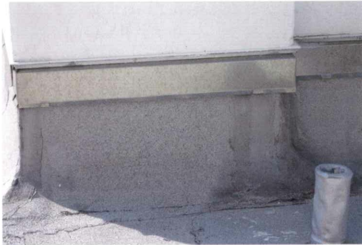
Stainless Steel Counter Flashing (Proper Height)
