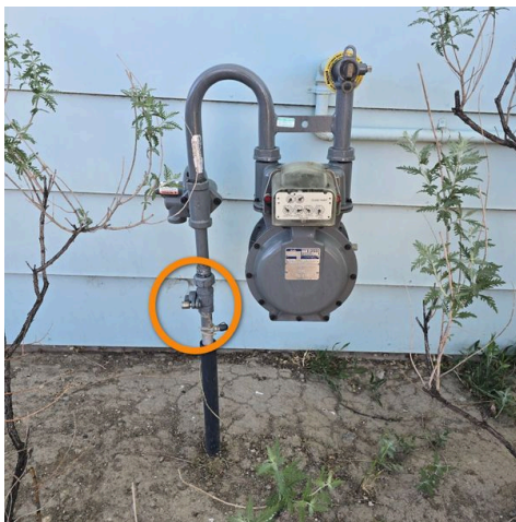
Gas Valve OFF and LOCKED at the time of the inspection. Close Up View
