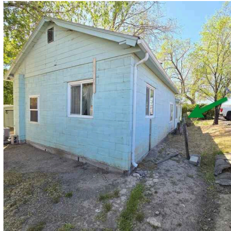
Gas Meter Location
