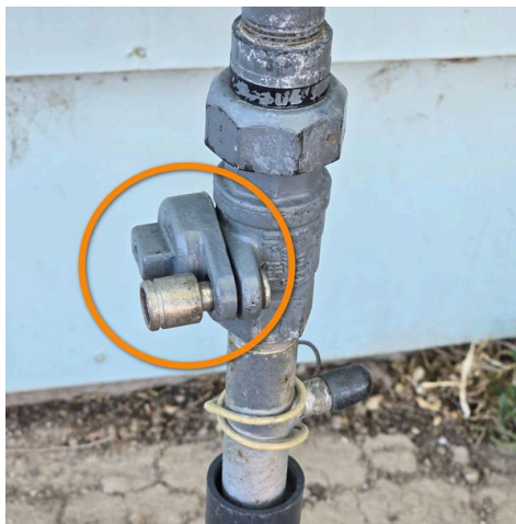
Gas Valve OFF and LOCKED at the time of the inspection. Close Up View
