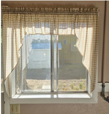
Aluminum Framed, Single Pane Example
