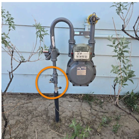
Main Gas Valve OFF at the time of the inspection
