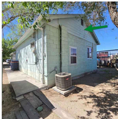
Exterior Access (no longer needed with interior ladder)
