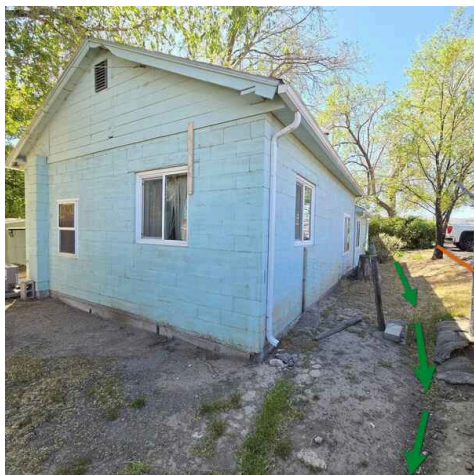
The adjacent lot is higher than the house. A valley has been dug to help water flow to the downhill (north) side of the lot.
