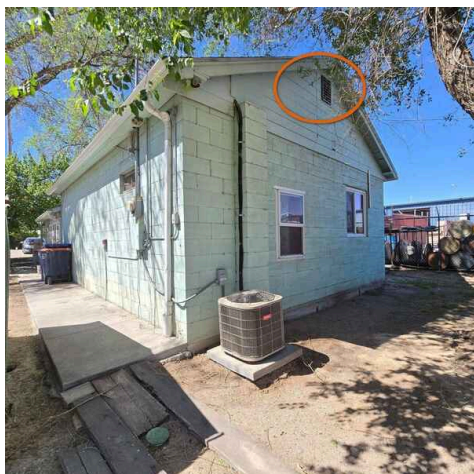
Gable Vents are covered with plastic in the Attic
