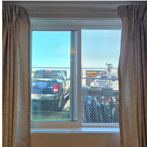
Vinyl Framed, Thermal Pane Example
