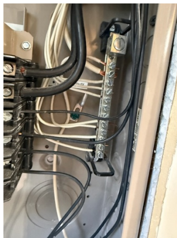
11.6.1 – Multiple neutrals under one lug. This was repaired by a licensed electrician. Surge Protection was moved to the top of the panel, and the panel was re-labeled.
