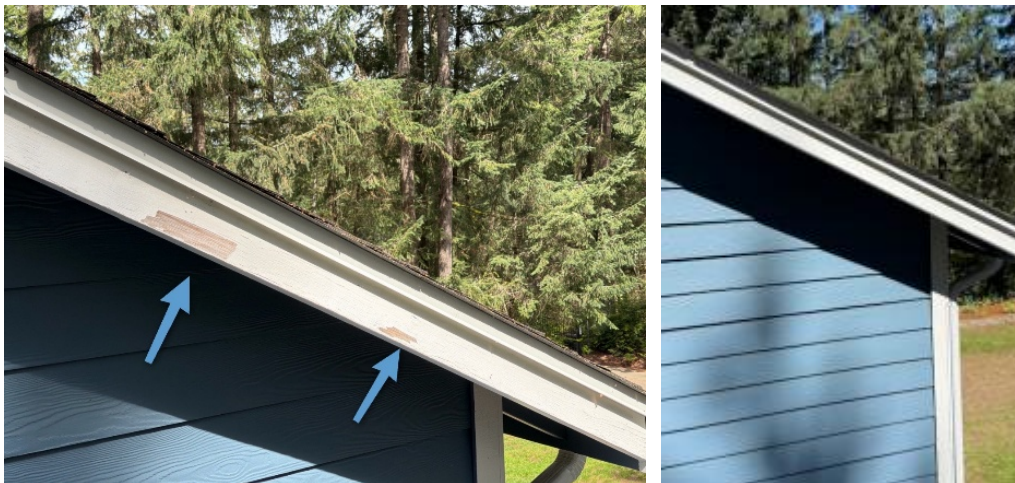
4.7.1 – Exterior Trim Paint. Trim was scraped and repainted.
