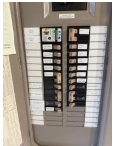
11.6.1 – Multiple neutrals under one lug. This was repaired by a licensed electrician. Surge Protection was moved to the top of the panel, and the panel was re-labeled.
