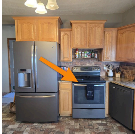
No Anti-Tip Bracket Installed
