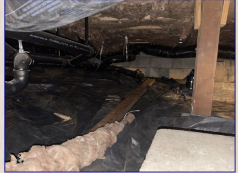
Vapor barrier present and properly installed.
