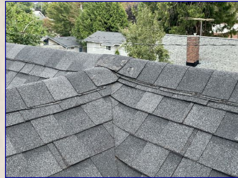
All exposed fasteners had been secured and sealant applied.
