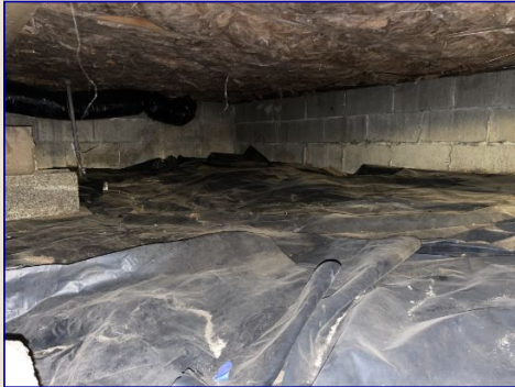
Vapor barrier present and properly installed.
