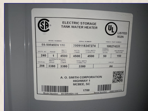
The Water Heater Data Tag
