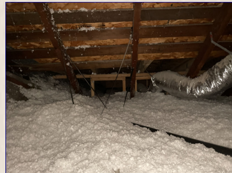
The Attic View
