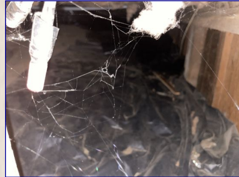
Vapor barrier present and properly installed.
