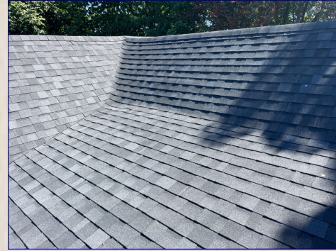
The Roof View
