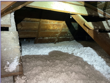
The Attic View
